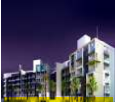
SHALIMAR ASHRAYA Kankanady, Mangalore
